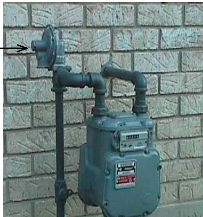
FIGURE 2 - GAS REGULATOR VENT
